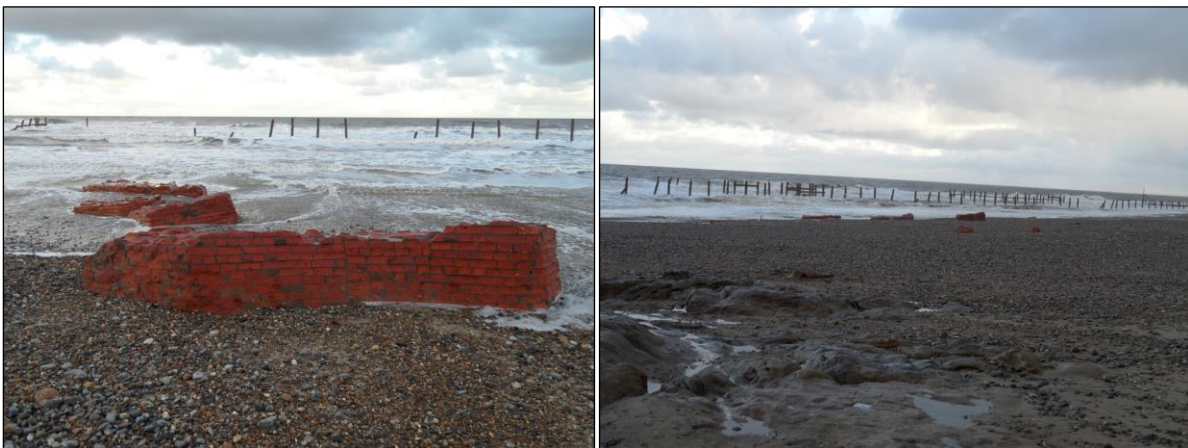
Plate 17.1 Potential remains of Happisburgh Low Lighthouse observed during site visit
